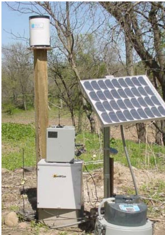
A 674 rain gauge connected to an Isco 6712 or Avalanche sampler is ideal for collecting rainfall data as well as runoff-triggered samples at remote monitoring sites.
